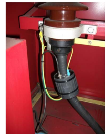
Inductive coupling in MV lines, courtesy of RSE
