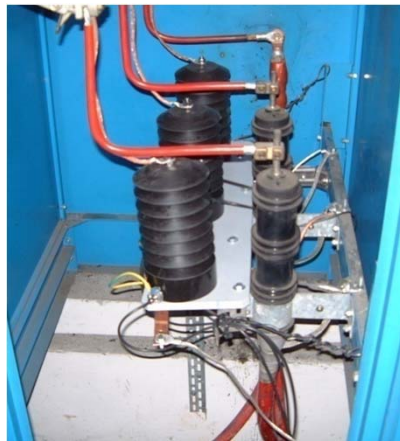
Capacitive coupling in MV lines, courtesy of RSE
